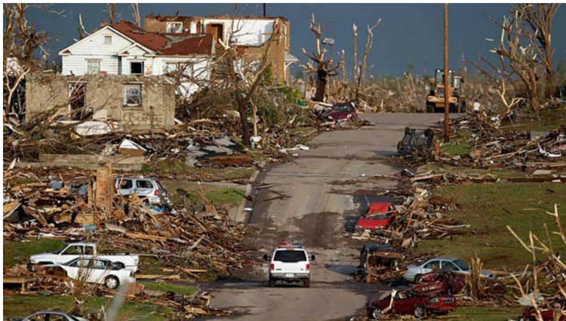
FIGURE 1.2 Tornado damage in Joplin, Missouri, from the May 2011 tornado that struck the area, killing 159 people and injuring more than 1,000 others. The tornado was the single deadliest in U.S. history since such records have been kept. The tornado was one mile wide and traveled 22 miles on the ground (NOAA, 2011). Source: Charlie Ridel/AP Photo
