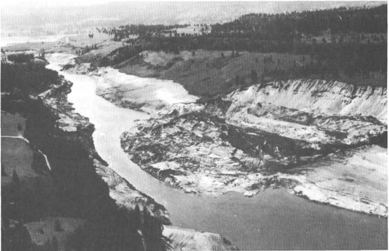
Figure 18. Jackson Springs landslide on the Spokane arm of Franklin D. Roosevelt Lake, Washington, 1969. This landslide was triggered by extreme drawdown of the lake (photograph by the U.S. Bureau of Reclamation).
