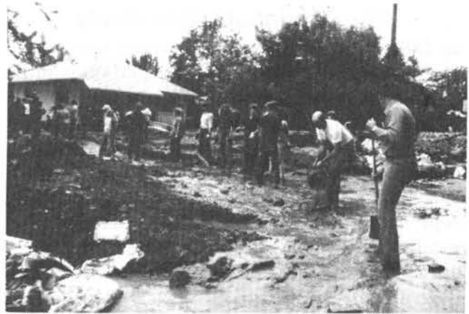
Figure 3. Local volunteers form "bucket brigade" to help clean mud and debris from homes in Farmington, Utah in 1983 (photograph by Robert Kistner, Kistner and Associates).
