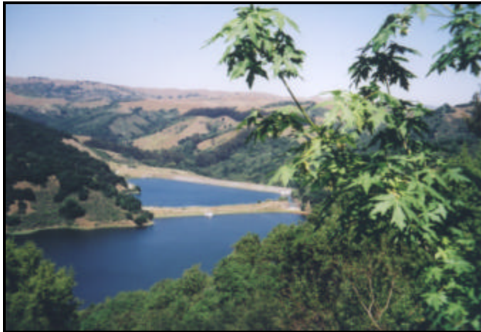
Upper San Leandro Reservoir showing original hydraulic fill dam and newer replacement dam
