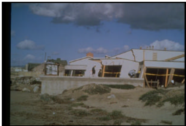
1989 Loma Prieta Earthquake – Moss Landing Marine Laboratories Showing structure “stretched” more than 5 feet due to lateral spreading
