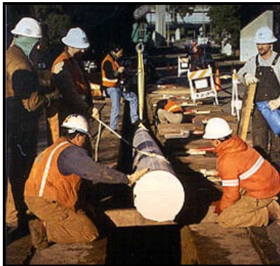
Gas pipelines being replaced in San Francisco Source – W. Savage, PG&E
