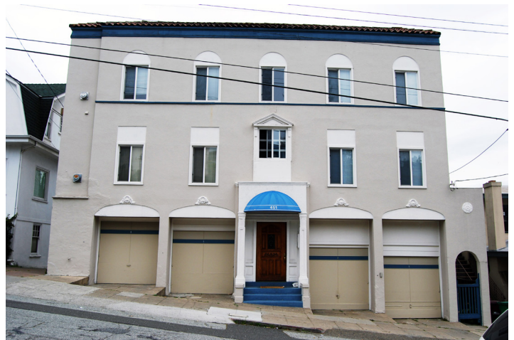
Potential soft-story apartment building in Oakland's Lake Merritt neighborhood.
